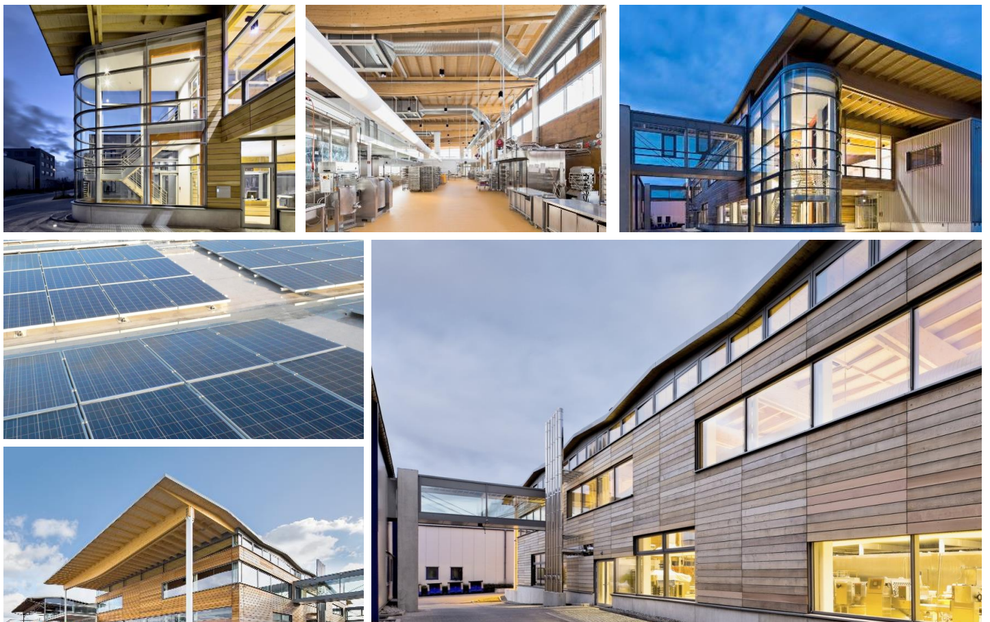
Figure 2.05: Architectural impressions wooden structure and envelope, solar roofing (source: Peter Bakery Essen, Germany, Phase 2, RMA Architects)
